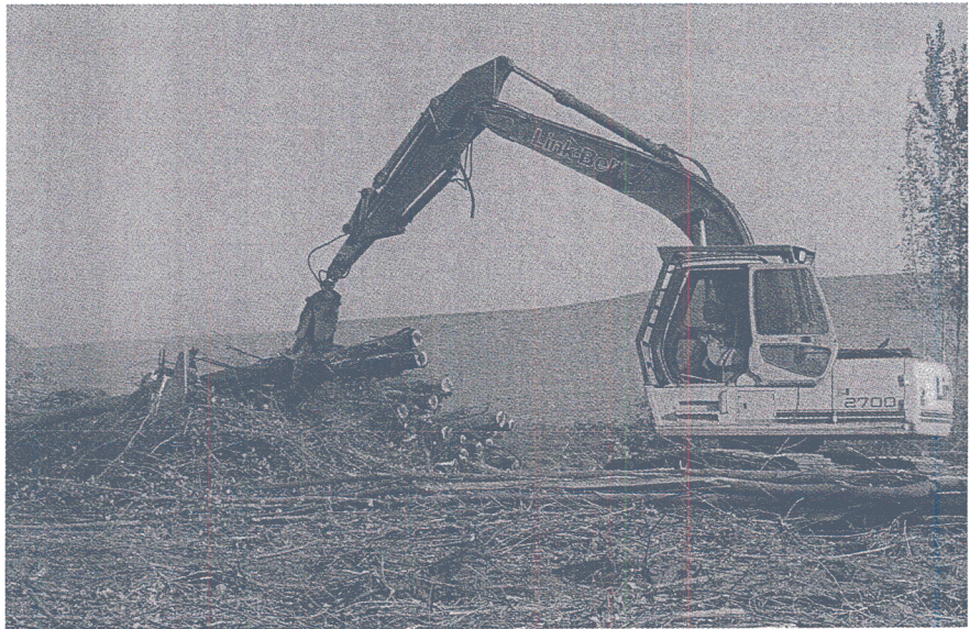
Figure 4. — Link Belt excavator with grapple, pulling trees through the Danzco delimeter.
